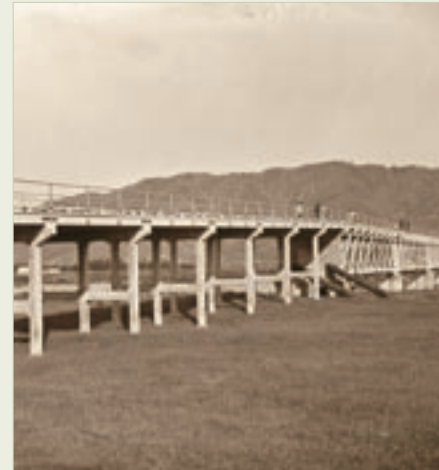
The 1909 pipe bridge on the Hutt River carried water from Wainuiomata to Wellington for 45 years. (A P Godber Collection, Alexander Turnbull Library, Wellington, NZ. Reference G-453-1/2-APG)
