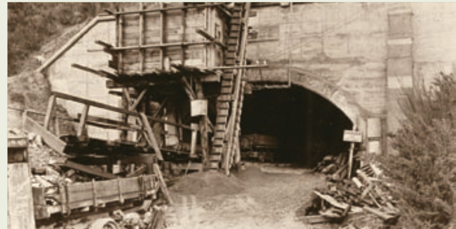
The road tunnel project to link Wainuiomata with the Hutt Valley was abandoned in the 1930s (shown here), but produced dividends when in 1981 it was finished in a smaller bore for water pipes. (Alexander Turnbull Library, Wellington, NZ. Reference F-65767-1/2)
