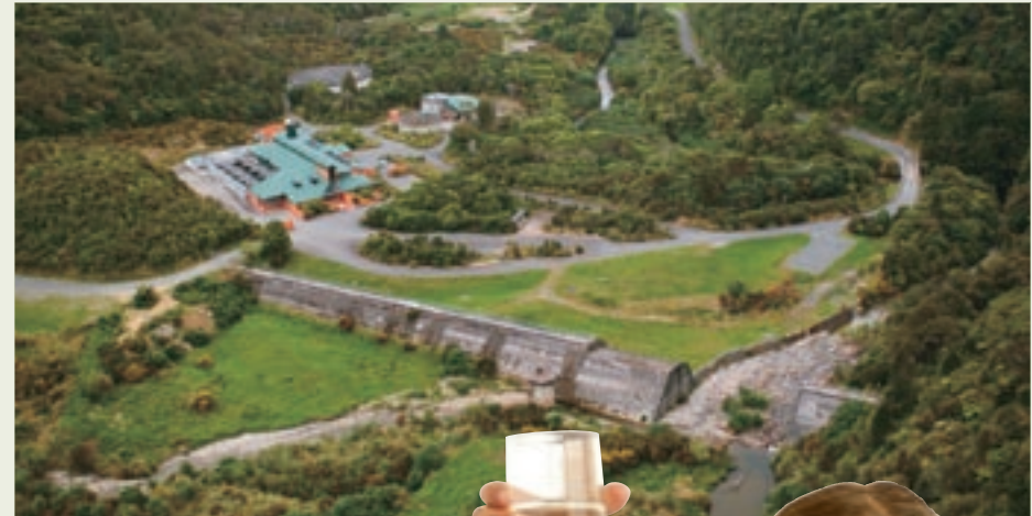
The Wainuiomata water treatment plant, with its state-of-the-art treatment process, was opened in 1993. The decommissioned Morton Dam can be seen in the foreground.
