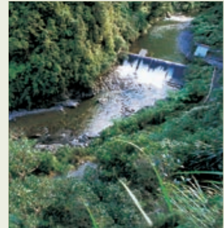
The water intake at Kaitoke on the Hutt River, seen here under construction (September 1952, left) and complete (above). Building the intake proved challenging, as it is situated in a narrow gorge that is subject to flash floods and the river could not be diverted away from the construction site.
