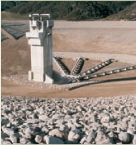
The smaller of Te Marua's twin lakes ready for filling. The radiating inlet pipes at the base of the tower help circulate the stored water.
