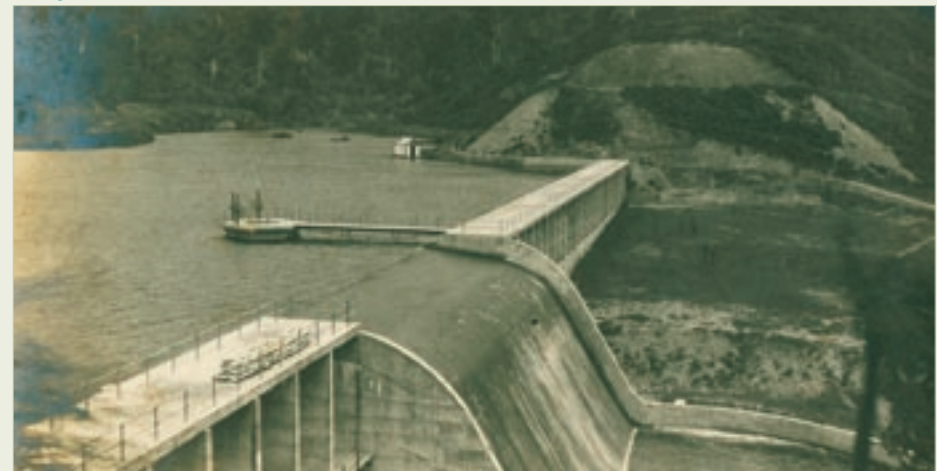
Morton Dam was named after William Morton, the city engineer who oversaw its construction. It was a concrete buttress dam and its cellular mode of construction was 'state of the art' at the time. The spillway was removed when the dam was decommissioned in 1988.
