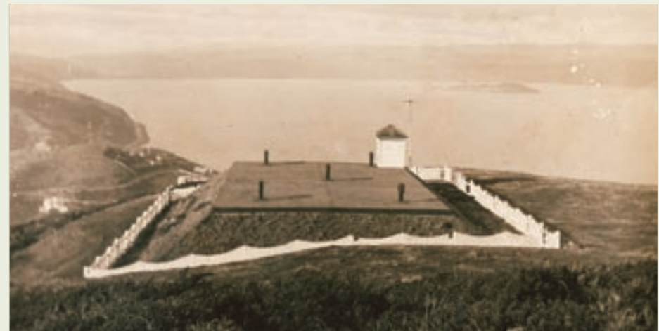
Wellington's high peaks were used for several service reservoirs, to which water had to be pumped, but which then gave a good gravitational flow to residents. This is Wadestown's reservoir, 241 metres above sea level, built in 1911 and smartly fenced.
