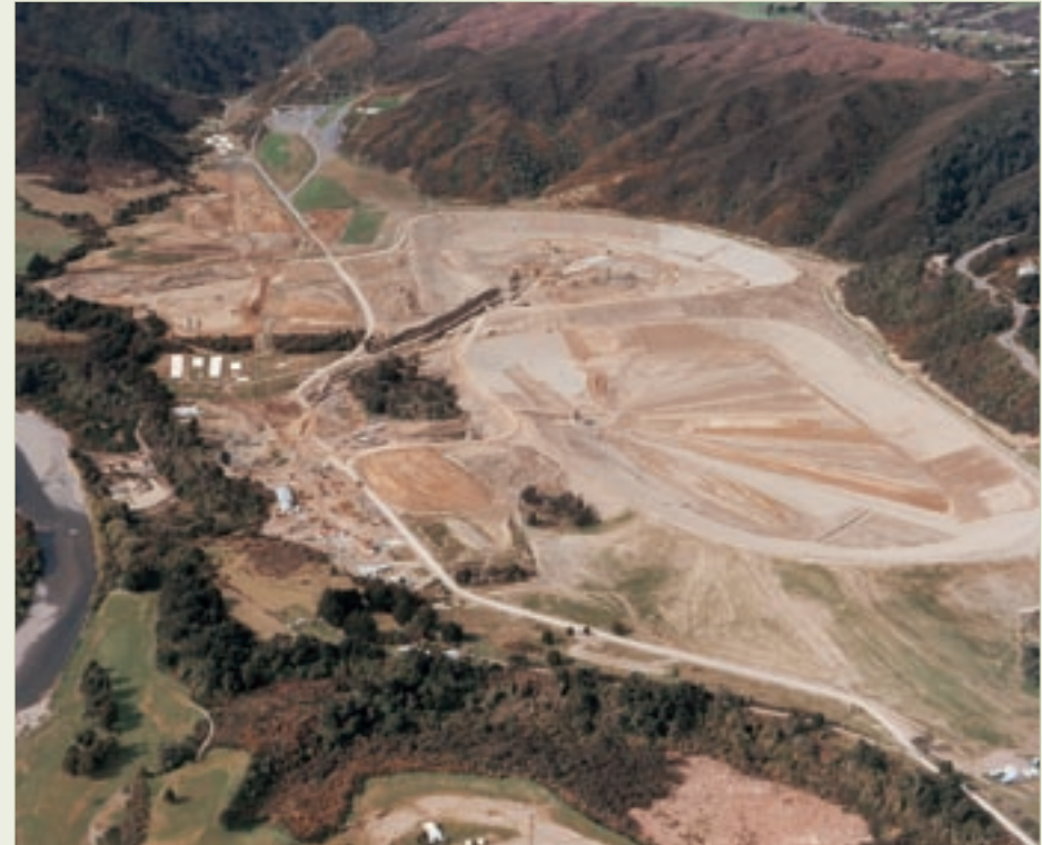
The 'moonscape' of the Te Marua twin lakes construction site, September 1983.
