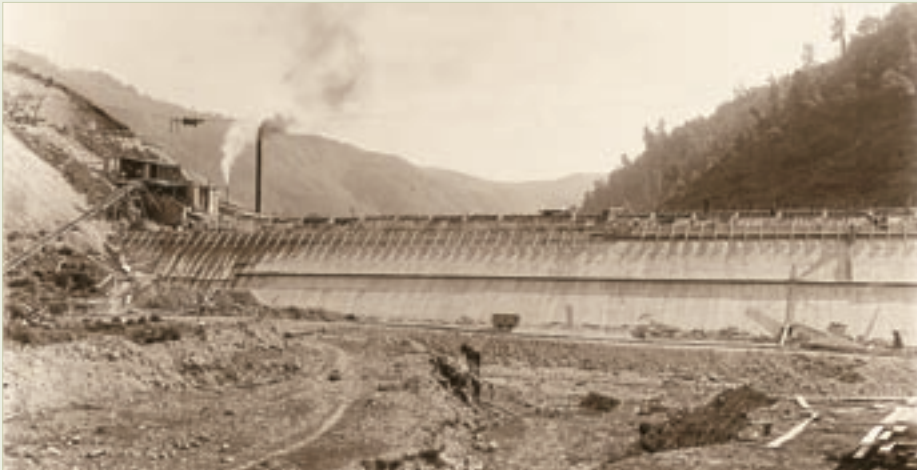
The second Wainui dam (Morton Dam) under construction beside Solomons Knob in Sinclair Valley (circa 1911). (S C Smith Collection, Alexander Turnbull Library, Wellington, NZ. Reference G-20074-1/1)
