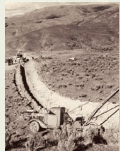
Laying of the Porirua branch line off the Kaitoke-to-Karori water main. (The Dominion Post, Wellington, NZ)
