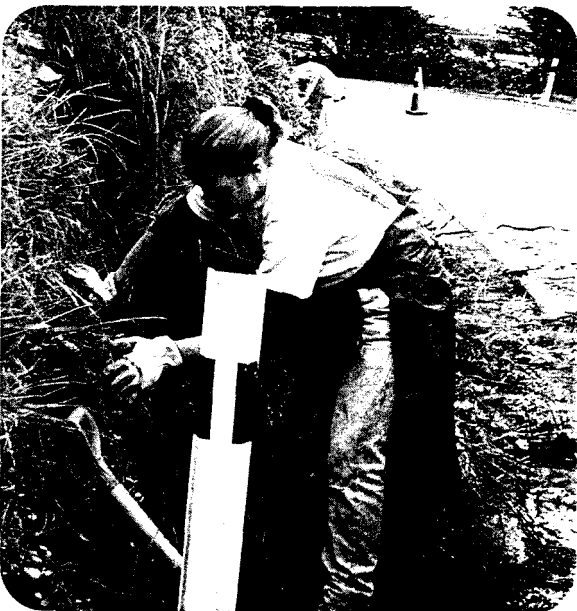
Digging at the excavation site on Henderson's Bend, SH58 as part of the Pauatahanui Bridge Replacement project
