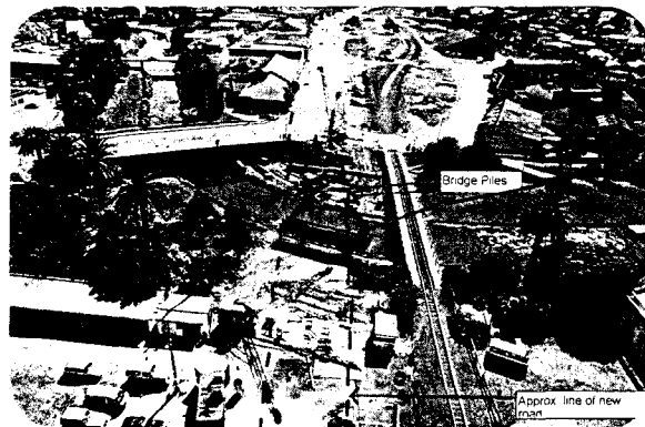
The new bridge currently under construction over the Taylor River
