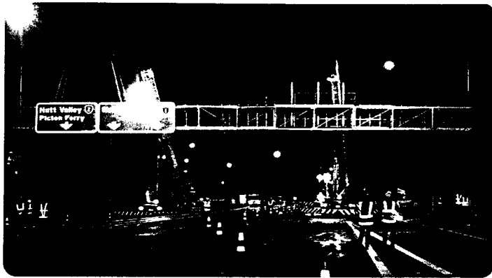
Installing part of the active traffic management system (ATMS) along Ngauranga Gorge
