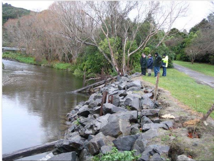
Figure 1 Poole Cres Rockline Looking upstream
