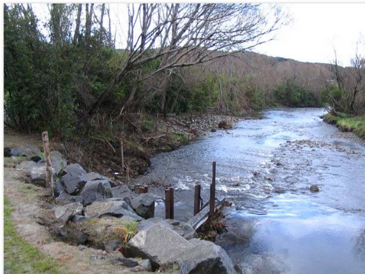
Figure 2 Poole Cres Rockline Looking downstream
