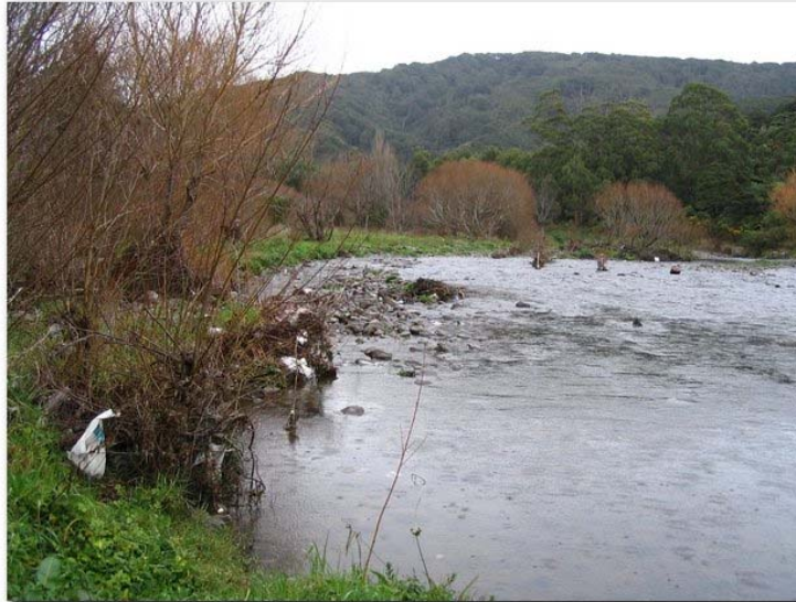
Figure 3 Looking Downstream - out flanked poles and over wide bed
