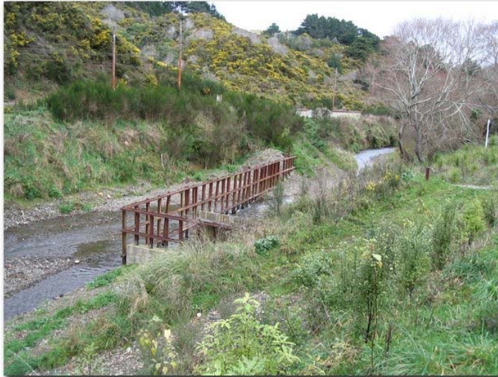
Figure 7 Debris arrestor looking upstream
