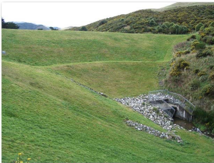
Figure 8 Down stream face of Stebbings dam
