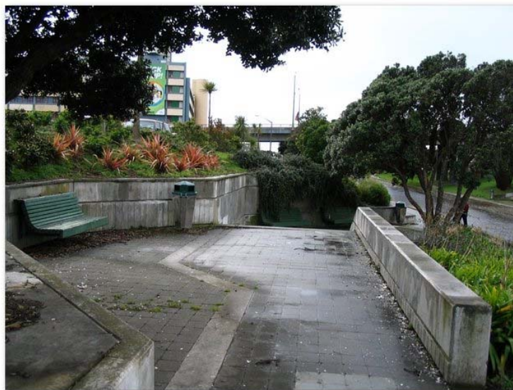
Figure 5 Flood wall incorporating seats and gardens
