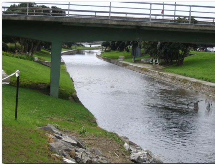
Figure 4 Cleaned out stream looking downstream
