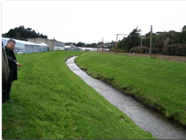
Figure 6 Looking down stream
