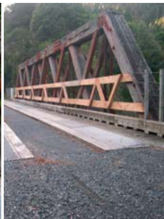
and after handrail installed
