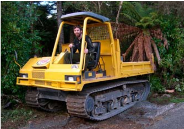
A gantry assisted with the Orange Hut toilet installation
