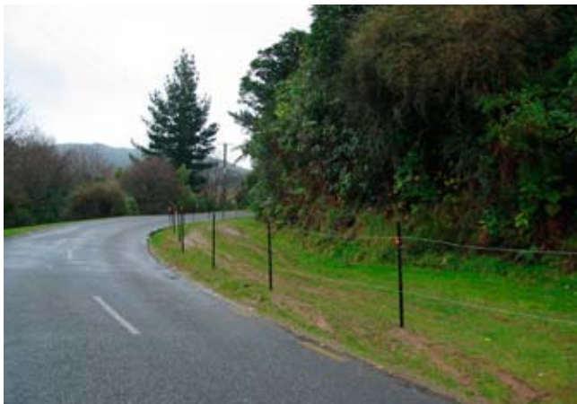
A temporary fence was put in before...
