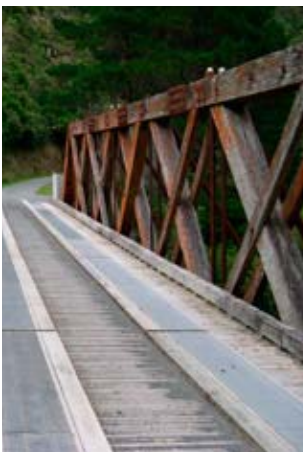
Pakuratahi Truss Bridge before handrail...
