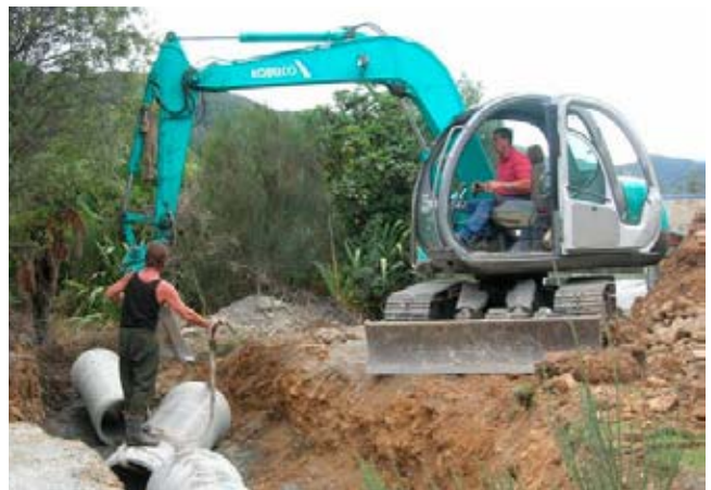
Tunnel Gully culvert pipes were upgraded
