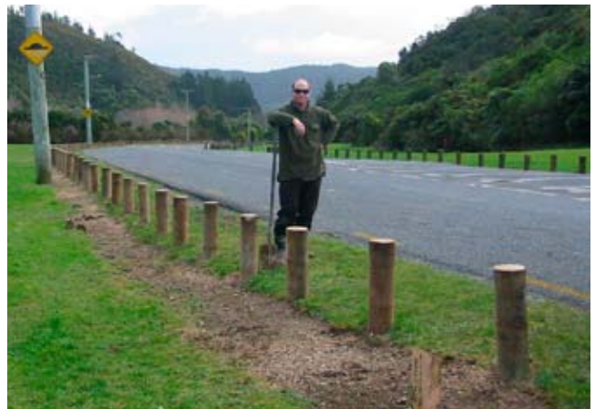
more permanent bollards were installed
