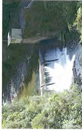
Kaitoke Weir: increased water take is being investigated
