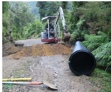
New culvert pipe on the Orongorongo Road
