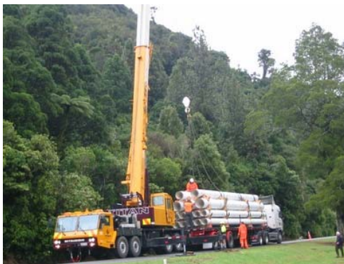
Unloading pipes for the seismic repair stocks
