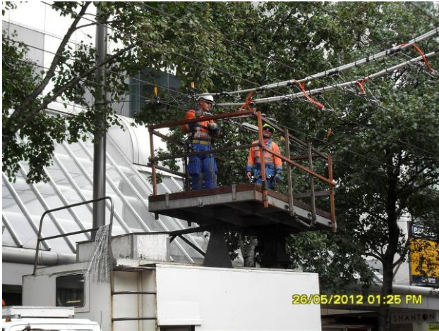
Installation of bus frequency counter
