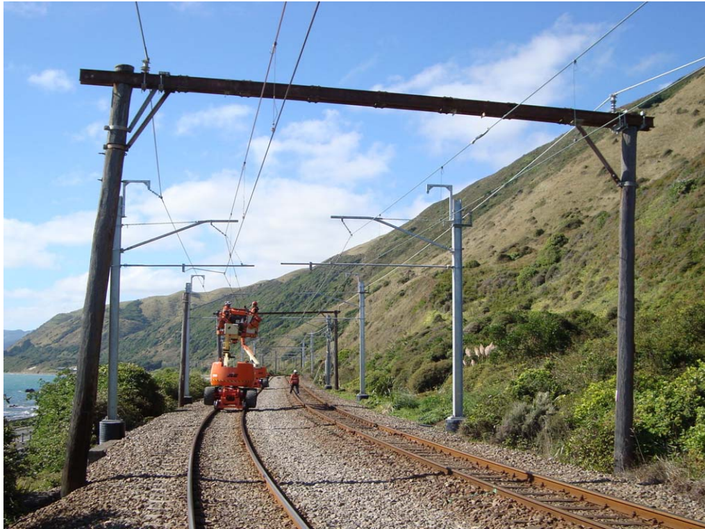
Work under way during March on the North Junction - Paekakariki section of the traction renewal project. The overhead wire is being transferred from existing life expired wooden/steel portal poles to the new steel cantilever structures.
