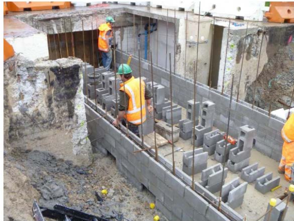
Installation of blockwork for the new staircase
