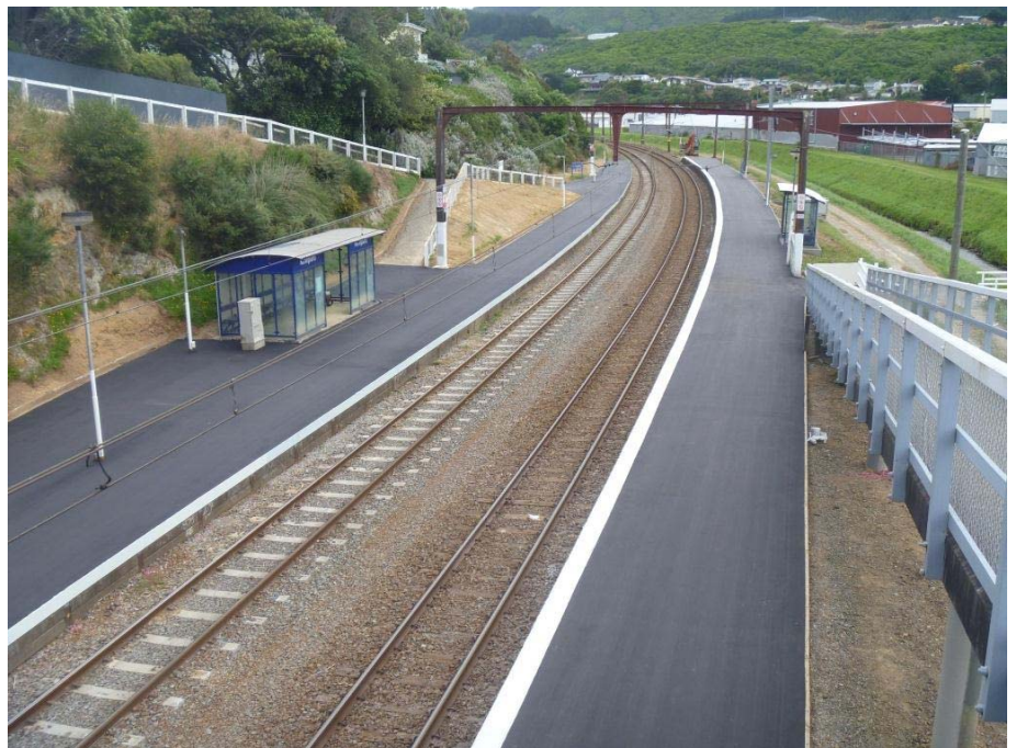
Kenepuru station with life extension works nearing completion
