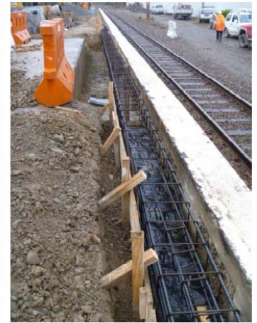
The reinforcing for the concrete capping beam at the north end
