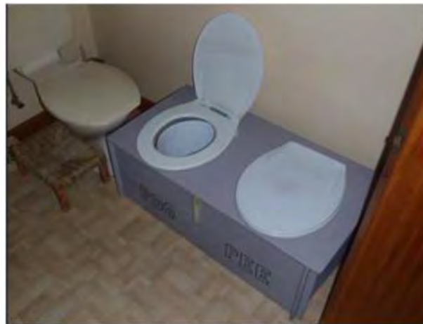
Photo 1: The two-chamber toilet box
