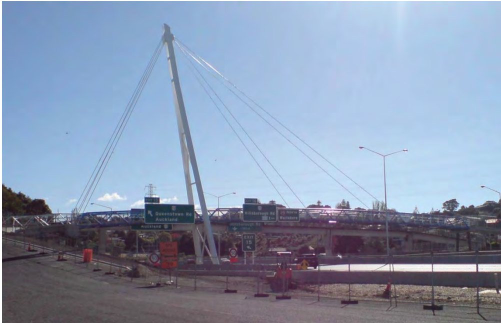
Figure 17: Beachcroft Avenue Footbridge SH20 - Auckland (NZTA)
