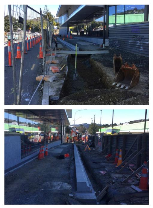
Preliminary work at Karori Stop A in order to facilitate the service relocations and the removal of the utility pole is complete. The construction at the main bus stop will commence shortly with completion expected to be late November.
