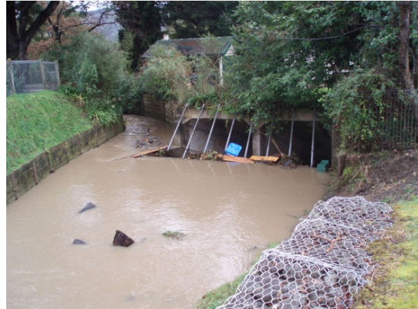
Figure 8 - Blockage forming at bypass intake
