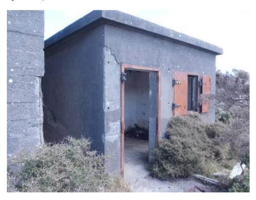
Figure 30: The wireless room. The reinforced concrete walls were rendered on the outside. The shutters are still in place and at the bottom of this photograph there is visible a small portion of the door which currently rests on the ground in front of the building.
