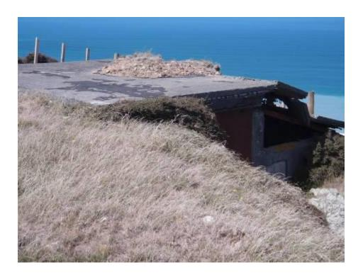
Figure 27: The observation post, built of reinforced concrete. Inside is the concrete foundation of what might have been a range finder or telescope. This building retains part of its camouflage (a layer of earth and vegetation visible on its roof) but the cantilevered roof over the viewing slit has collapsed. The path that has been constructed to allow entry to the building is shown to the right of the photograph
