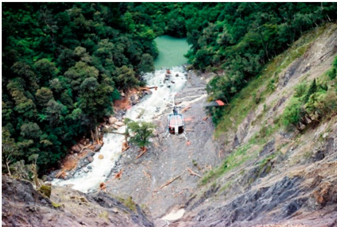
Figure 33: Major landslide and dam break in 1982 flood – GWRC.
