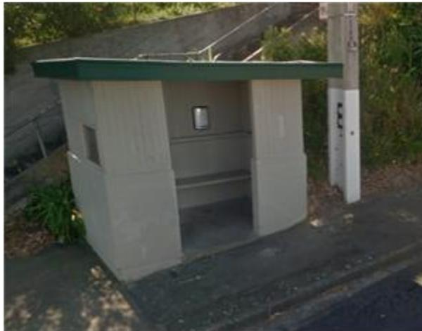
Figure 79: Concrete and wood bus shelter
