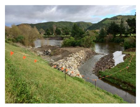
Figure 1: Site 1 Stokes Valley – Showing the stream diversion, with the weir repair area to the left of the photo
