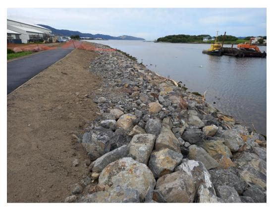
Figure 4: Site 11 Port Road, Seaview – Rock revetment and cycle trail
