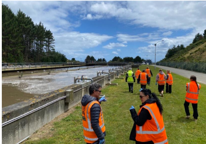
Figure 2. Accord partners at Porirua Wastewater Treatment Plant and outfall
